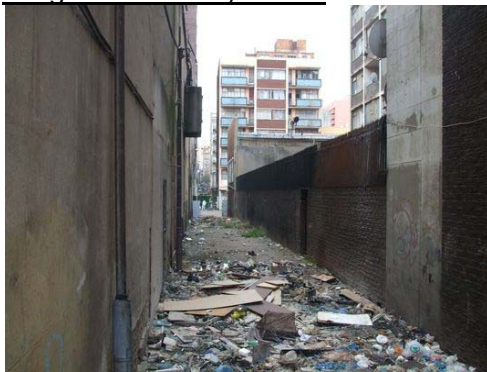
Image 2A: Lane 44 before upgrade
